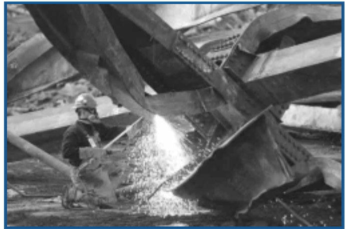
Ironworker cutting metal with a torch
