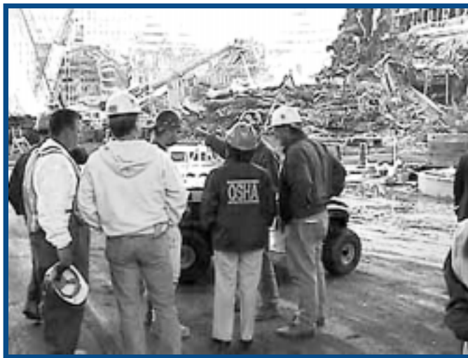
A partnership between the construction companies and OSHA called for all safety and health hazards to be voluntarily abated.
