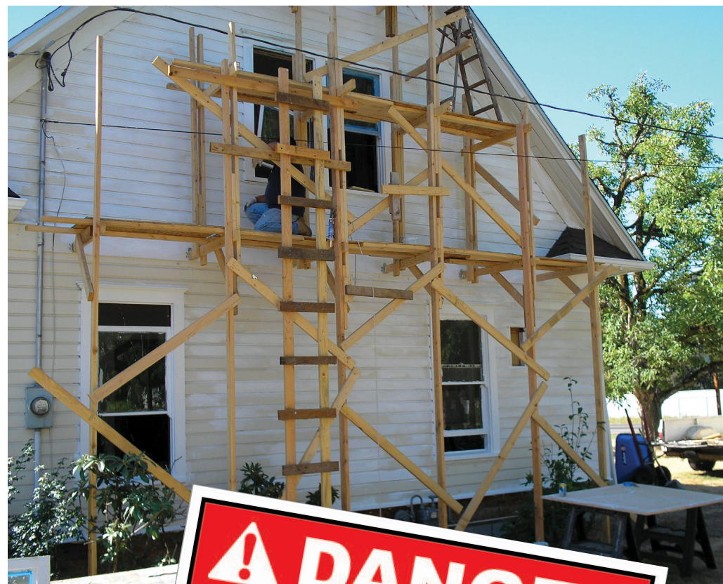
This worker is too close to the electrical lines!
