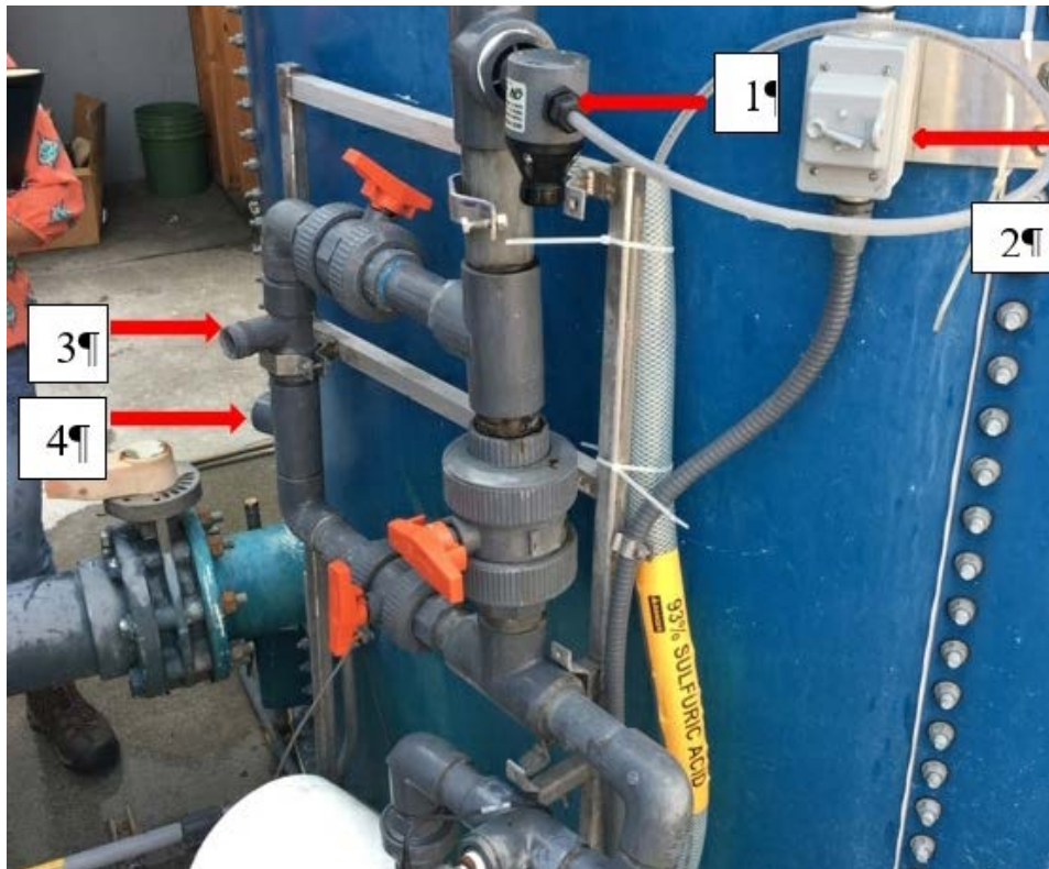
Closer view of the valves and pipe system associated with the pH tank: 1 is the acid injection point into the pH tank; 2 is the power switch to the acid pump shown at the bottom of the photo; 3 is where the pH probe was located in the system; and 4 is where the relief valve failed.
