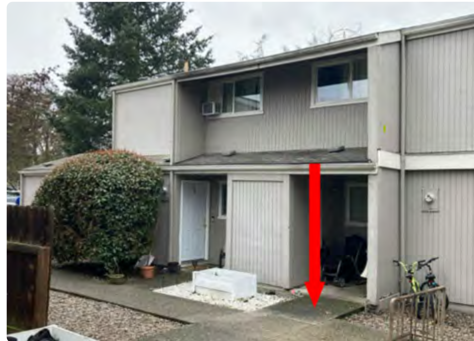
The employee fell 8 feet, 3 inches, while he was cleaning gutters on the first-story roof. (Source: OTIS, Image 0816)
